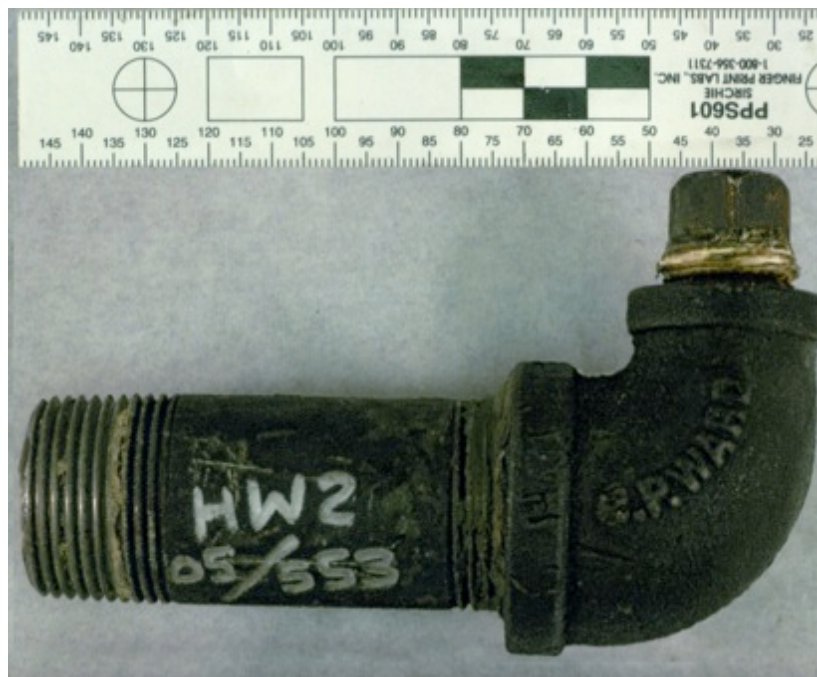
Photo 1-3 Pipe with tool marks.
