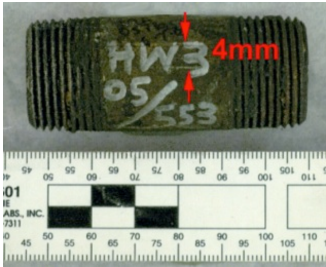
Photo 1-2 Pipe with tool marks. The spacing between tool marks on the pipe is 4 mm apart.
